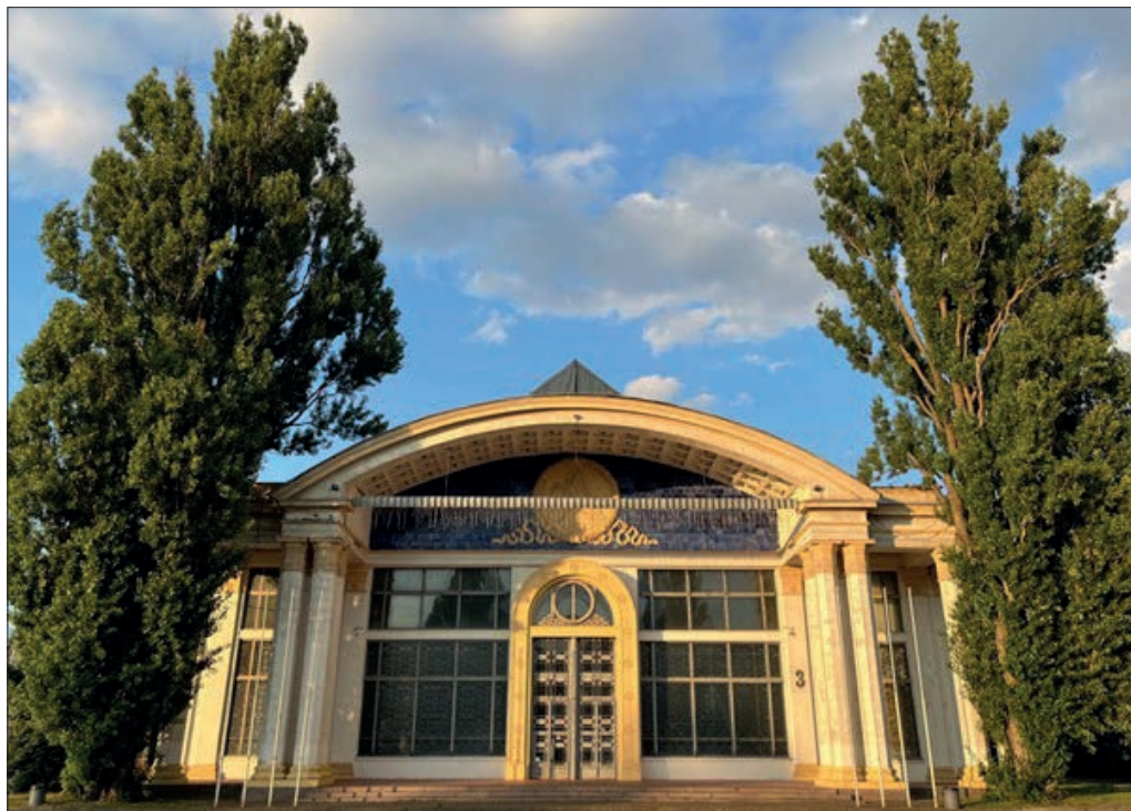
Fig. 8. Pavilion No. 3: Metallurgy. Architects: Mykhailo Hrechyna, Olena Mikhnevych, Mykola Hubov. Photo by Yevheniia Moliar
