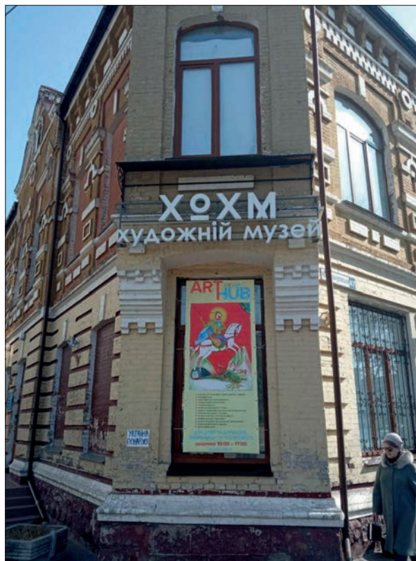
Fig. 17. The façade of KRAM building, Khmelnytskyi. KRAM_Art_Hub banner. 2022
