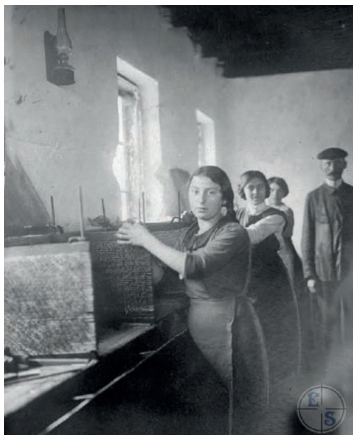
Fig. 22. Dipping frames at the Rivne Match Factory. Photos by Solomon Yudovin
