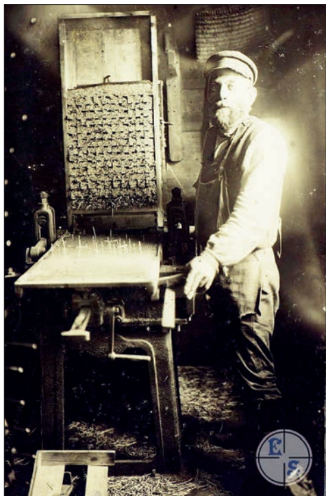
Fig. 19. A frame-filling machine at the Rivne Match Factory. Photo by Solomon Yudovin
