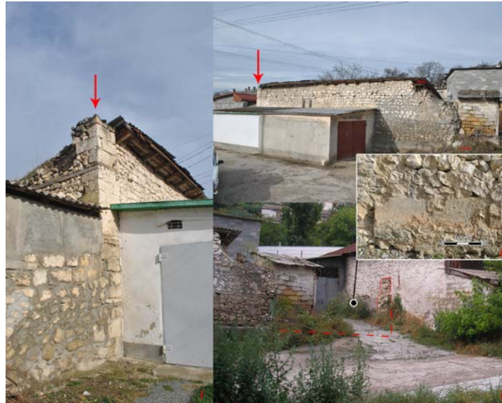
Fig. 9. Medieval wall in the building on Lenin street, 77 with its marking by red arrows
