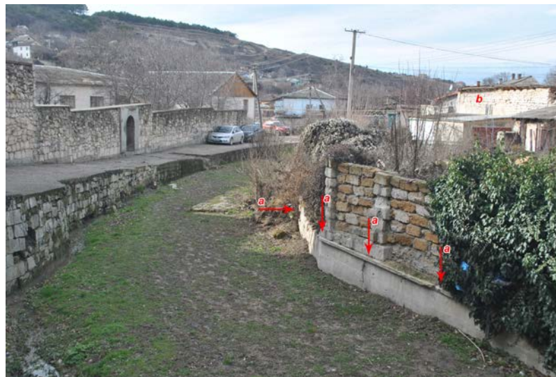
Fig. 8. The Churuk-Su river to the West from Embassy courtyard: a – the retaining wall of Churuk-Su riverbed; b - medieval wall in the building on Lenin street, 77
